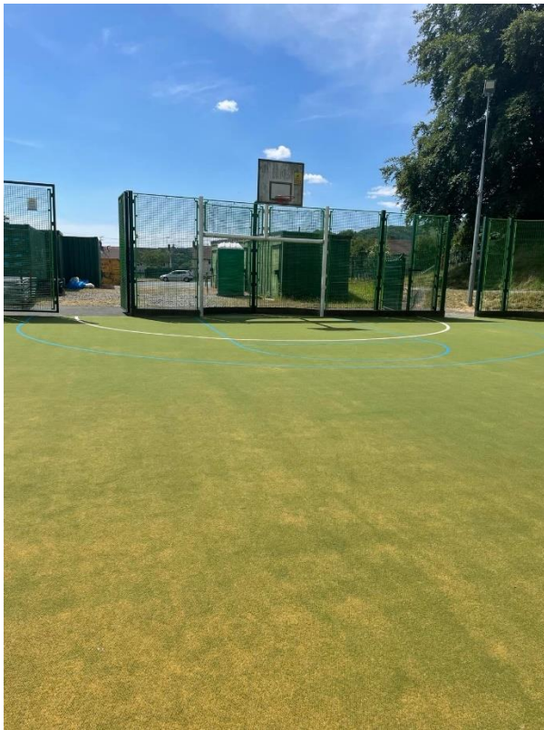
Pictures of the re-laid MUGA surface Plas Kynaston
